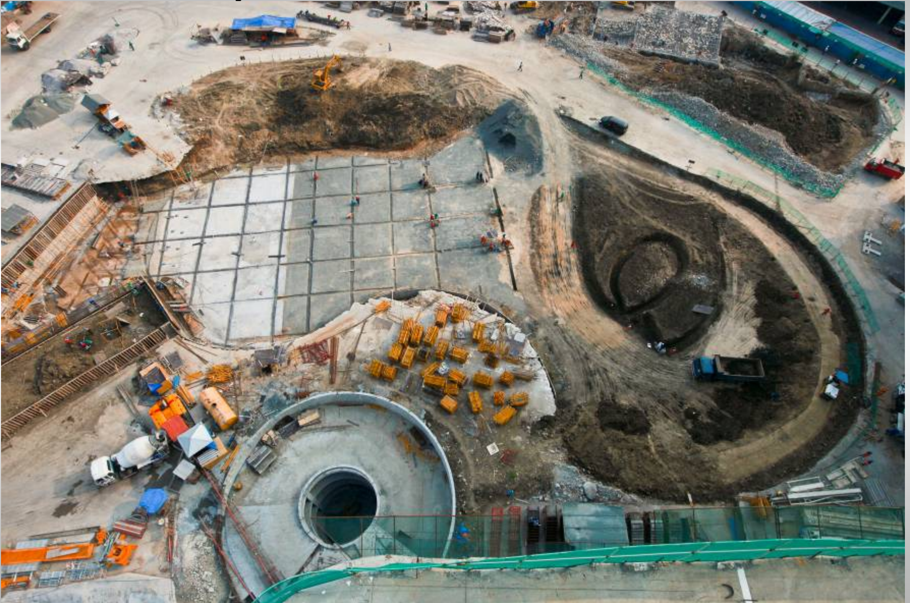
Construction works at the Azure's man-made beach
